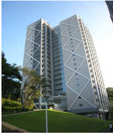
Figure 4-28 High-Rise Seismically Isolated Building (Building J2-3, Suzukakedai Campus)
