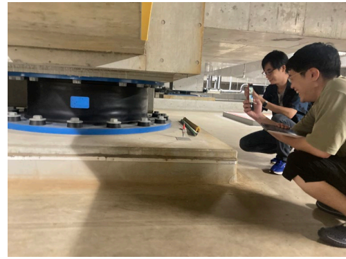
Figure 4-37 Tour of the seismic isolation layer of J2-3 building
