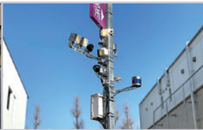
Road Side Unit (RSU)
